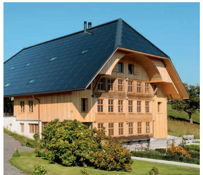
The frameless MegaSlate solar modules are laid just like conventional roof tiles. They are fitted by an authorized roofer or specialist installer.
