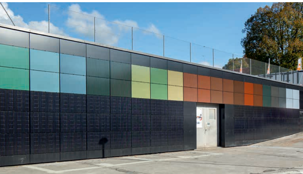
The use of state-of-the-art technologies such as colored or glare-free glass surfaces boosts public acceptance of photovoltaics in the building envelope.
