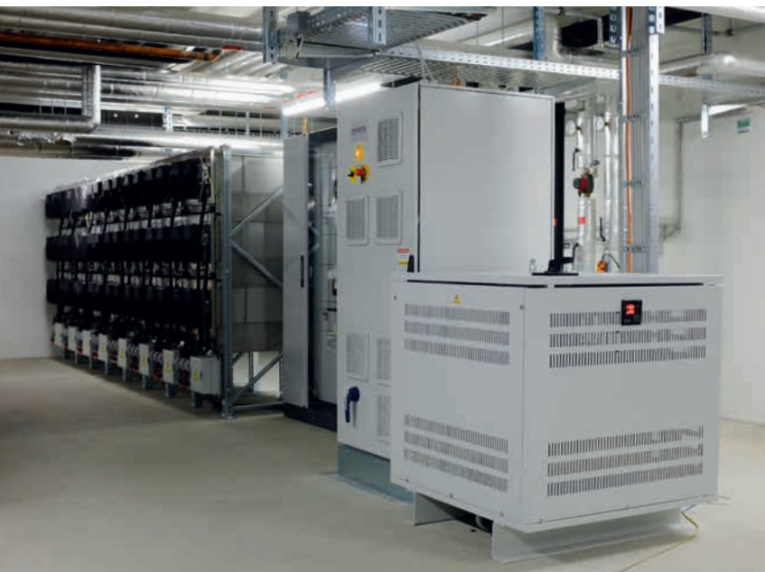
The salt energy storage facility at Migros in Schlieren (ZH) with a capacity of 540 kWh.
